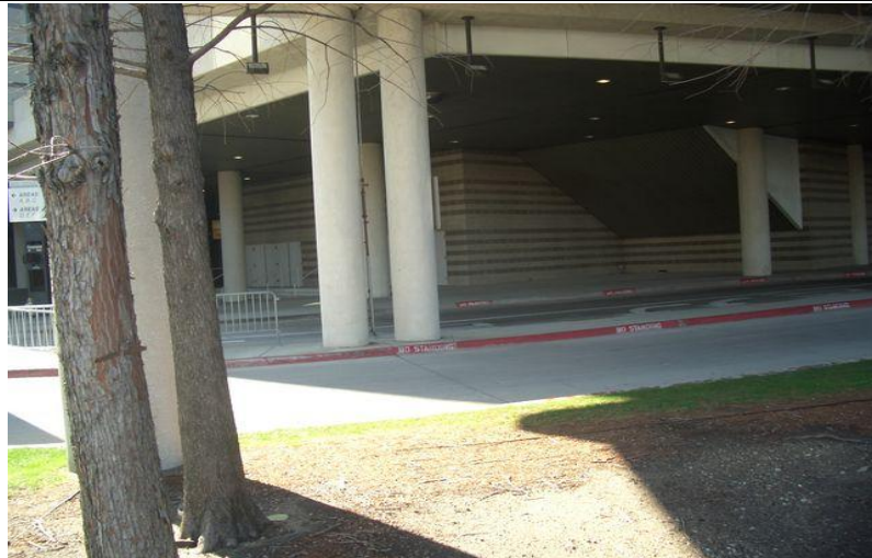
View from Site to the South
