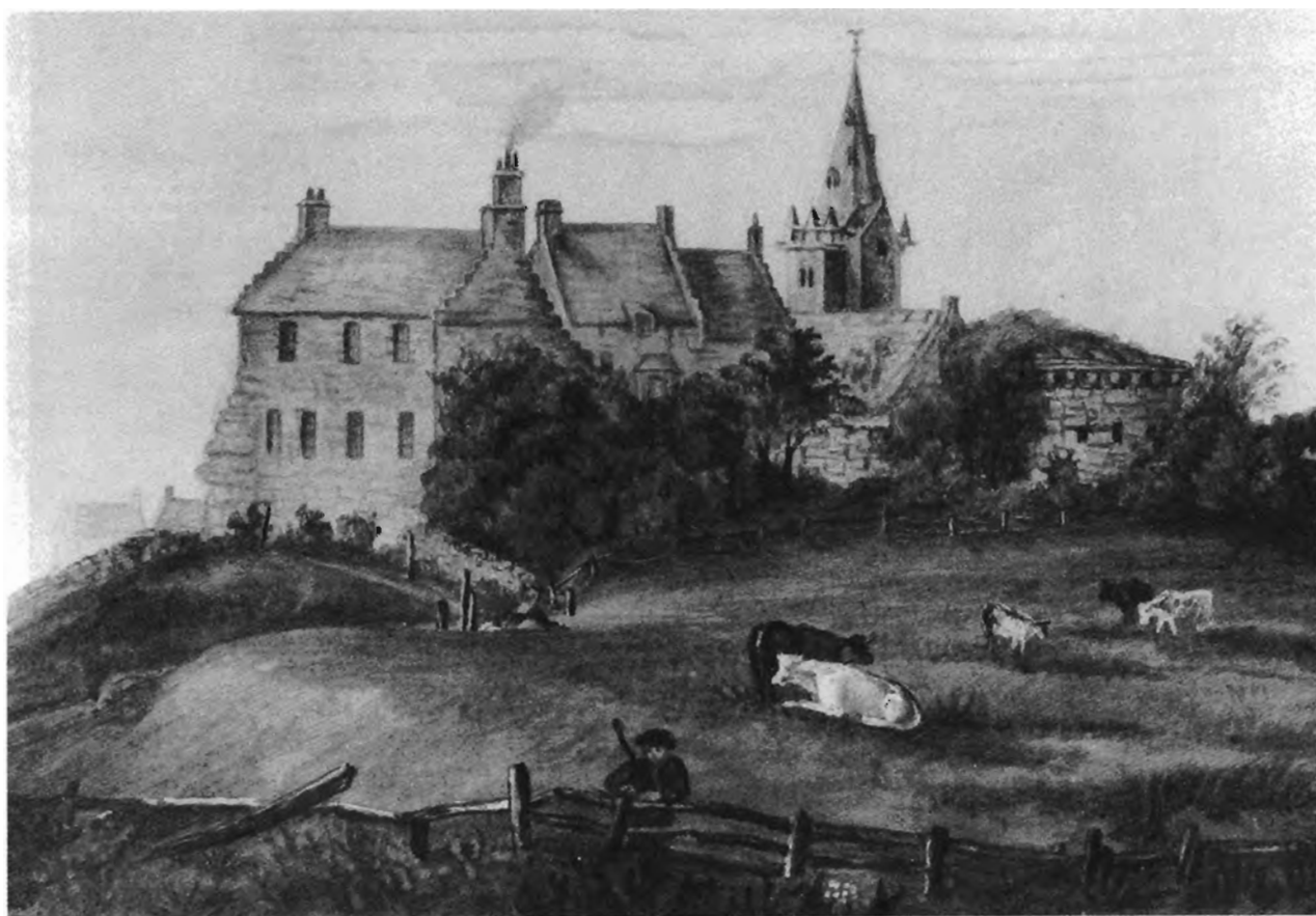
Illus 4.6. A detail from C E Horsburgh's watercolour, painted in 1818, of Pittenweem Priory. In the foreground, beyond the fence, the waggonway cutting is clearly seen. (Author's collection).
