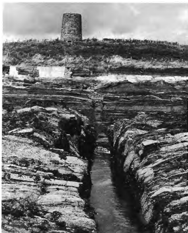
Illus 4.12. The rock-cut inlet channel at St Philips, looking north towards the wind-engine tower situated on the escarpment. The panhouses stood on the level ground immediately below it.
