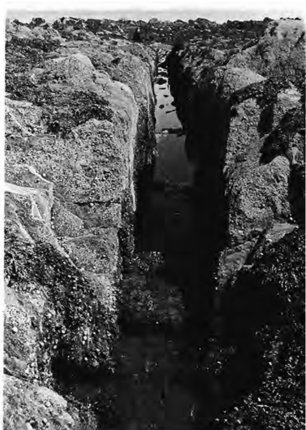
Illus 4.13. The inlet channel, looking seaward. The check for a sluice can be seen in the foreground.
