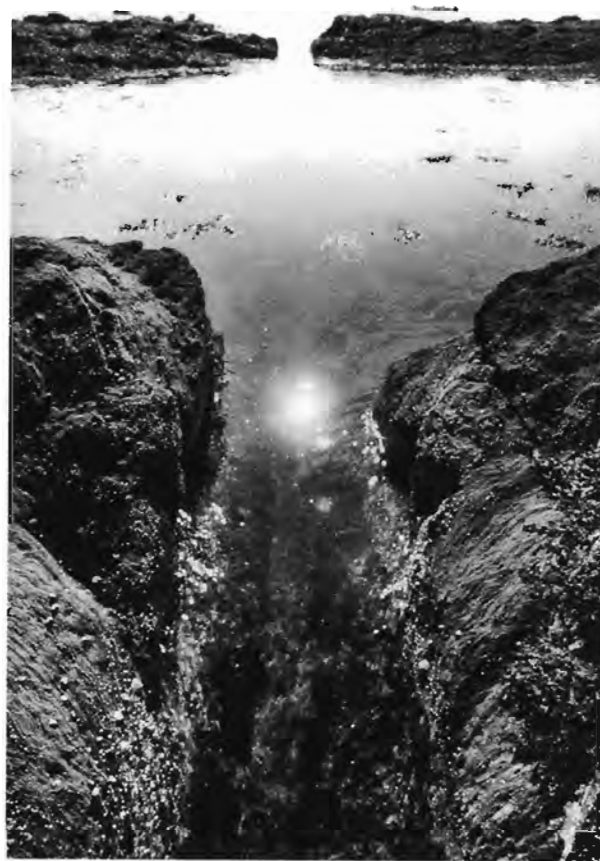
Illus 4.14. View across the reservoir as the tide flows in through the inlet channel (top). Note the U-section of the outlet pipe-channel in the foreground.
