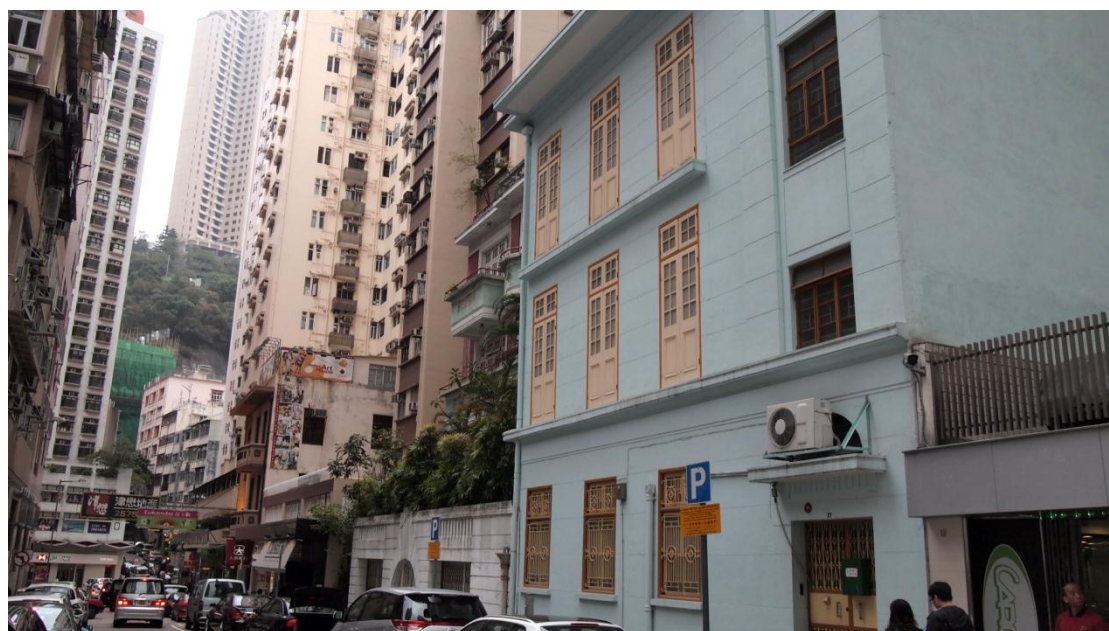
(FIGURE D5 No. 11, 15 & 17 Yuk Sau Street and No.54 Village Road)
