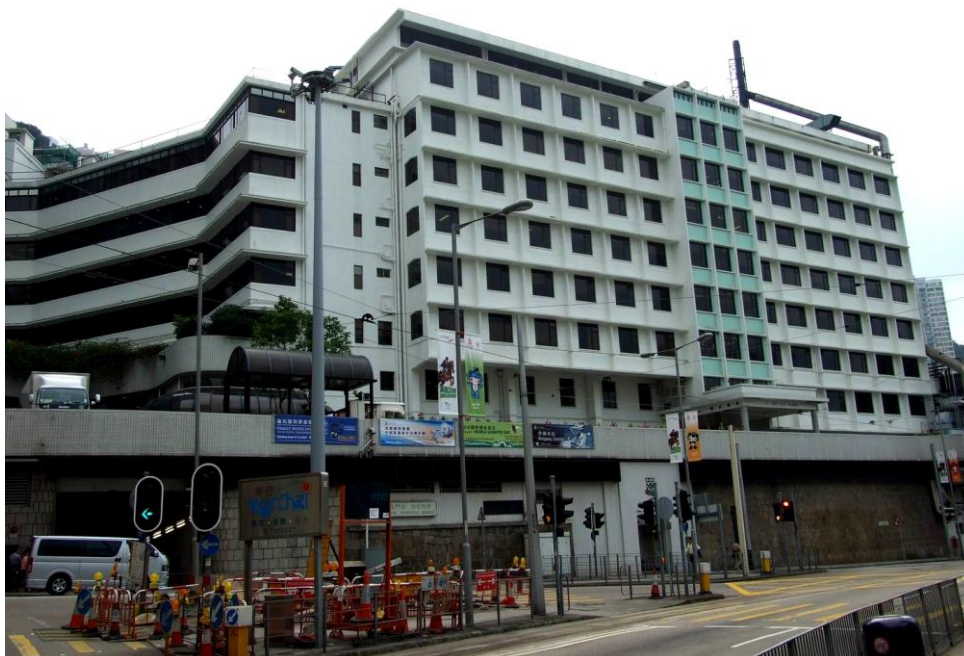
(FIGURE D9 The Hong Kong Sanatorium and Hospital [image from the online reference resources])
