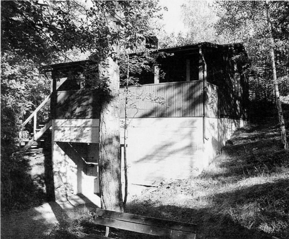
The entrance to the fort was disguised as a house. The entrance is through the fake 'garage doors' on the lower level. Photo by Dan McKenzie
