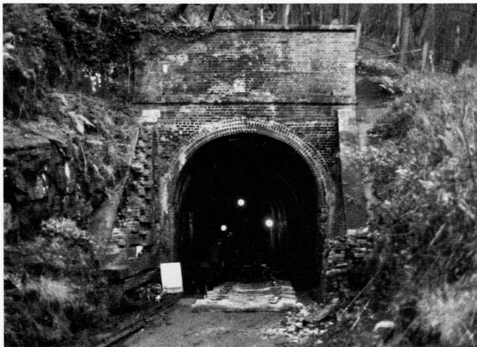
Berwyn Tunnel—East end
