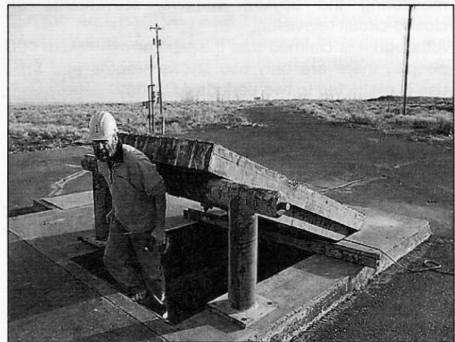
Bari Hotchkiss steps out of the abandoned former missile complex he owns east of Moses Lake. He has listed it on eBay.
