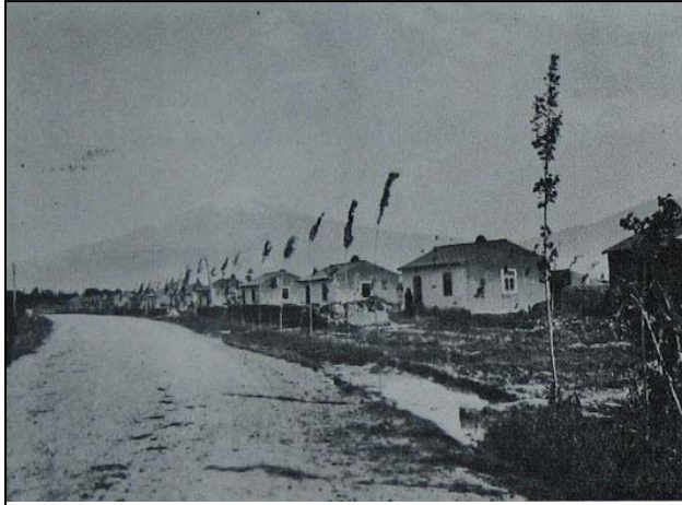
Photo 35: Newly built houses for settlers, 1935 (Birinci Genel Müfettişlik, 1939)
