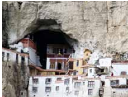
Structures set within the cave
