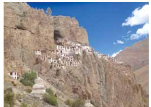
Structures of the Phuktal Gompa
