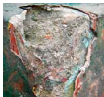
Thick layers of later additions
