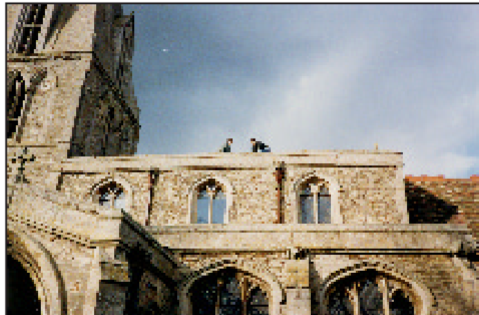
Fig. 4 John Burrows and Alan Hatfield repairing the church roof after gales
