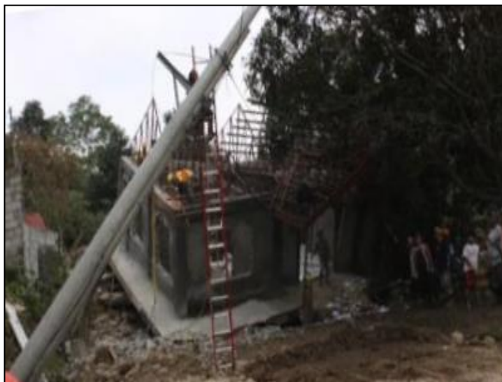
Destroyed house at the center of Naguilian-Baguio Road due to Rainfall-Induced Landslide caused by Typhoon Pepeng on October, 2009.
