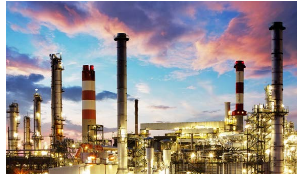
Dangote Refinery, Nigeria
