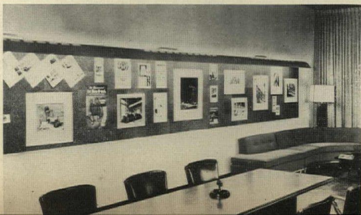
Wall lighting is more common in business conference rooms, as shown below, than in classrooms. This unit has rotating reflector, apertures for soft uplighting to reduce contrast.
