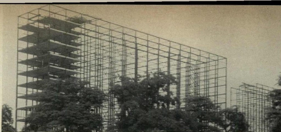
WELDED STEEL SKELETON frames group of apartment buildings in Paris. Some floor slabs are already in place.
