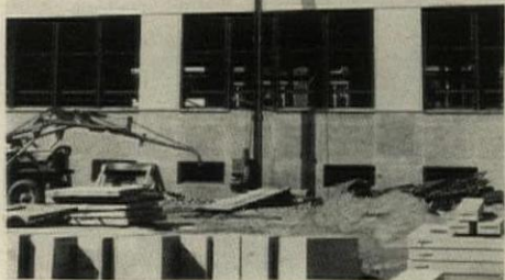
MONORAIL HOIST can lift one ton to any height desired by adding 6' sections.
