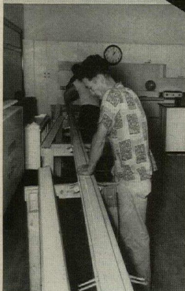
FIXTURES ARE PRE-ASSEMBLED AND PRE-WIRED AT FLOOR LEVEL
