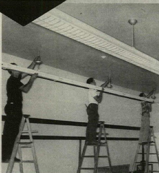
ENTIRE RUN IS RAISED TO CEILING AS A SINGLE UNIT
