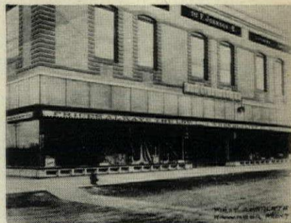
The first truly modern store front with large display windows in Kawneer resilient sash.
