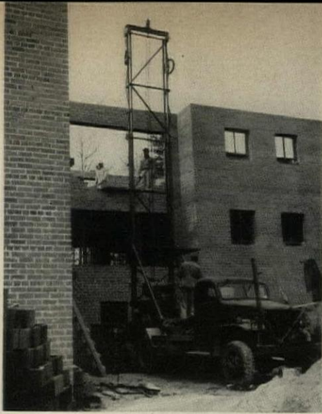
TRUCK-MOUNTED HOIST with 42' lift can be erected in less than half an hour.
