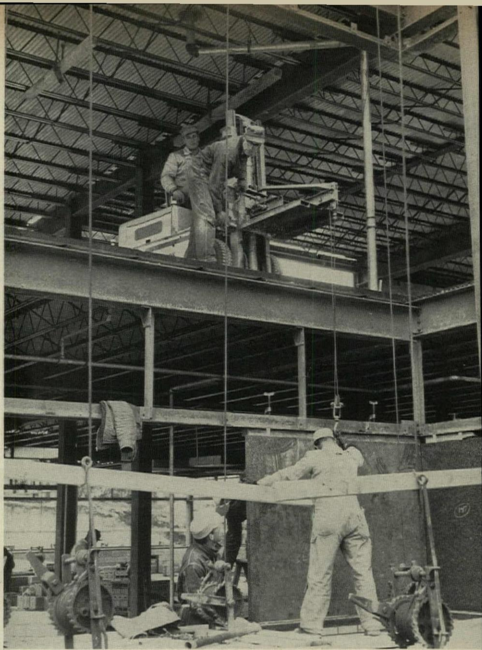
HAND-OPERATED WINCH added to fork truck doubles usefulness of machine.
