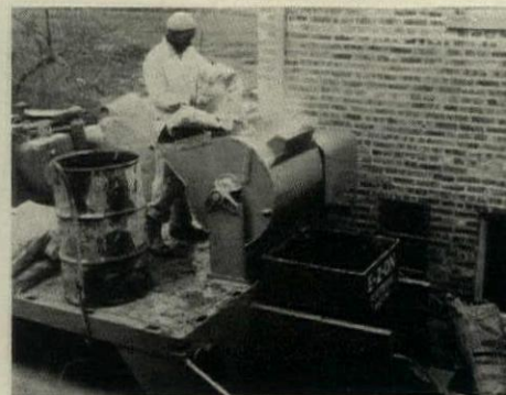
PLASTERING machine mixes, pumps and sprays on plaster at a saving of 50% in time.
