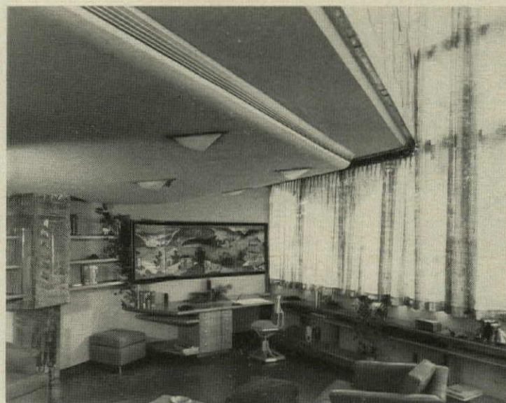
High ceilings enhance outer corners of living rooms; conditioned air is discharged from slots under mezzanine slab.
