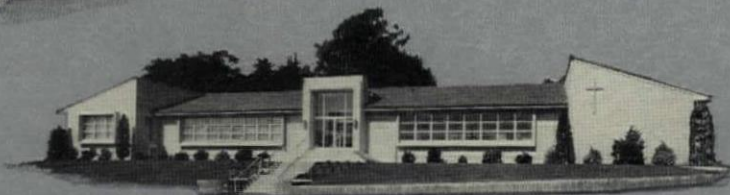
SPECIAL PURPOSE BUILDING Holy Cross Administration Bldg., Colma, Calif. Architects: Wilton Smith & John G. Minton Contractor: Ira H. Larsen Co.
