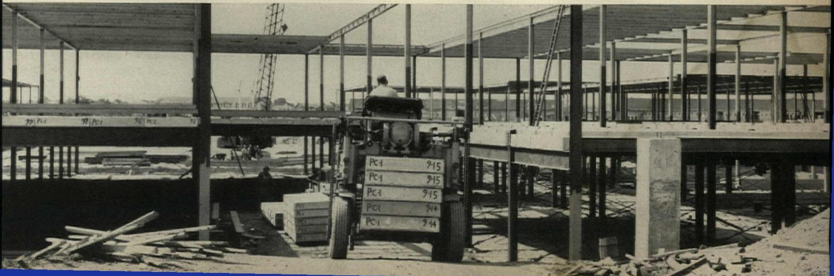
STRADDLE CARRIER (below) lifts and hauls precast slabs to a few yards of point of use.
