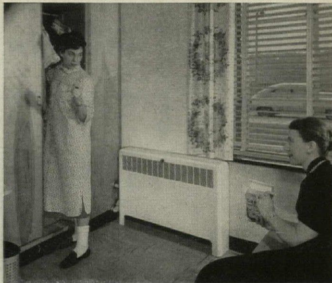
Dunham Convector in dormitory rooms... painted to blend with wall. Individual room heat control assured by knob-operated damper. Chain-operated damper available.
