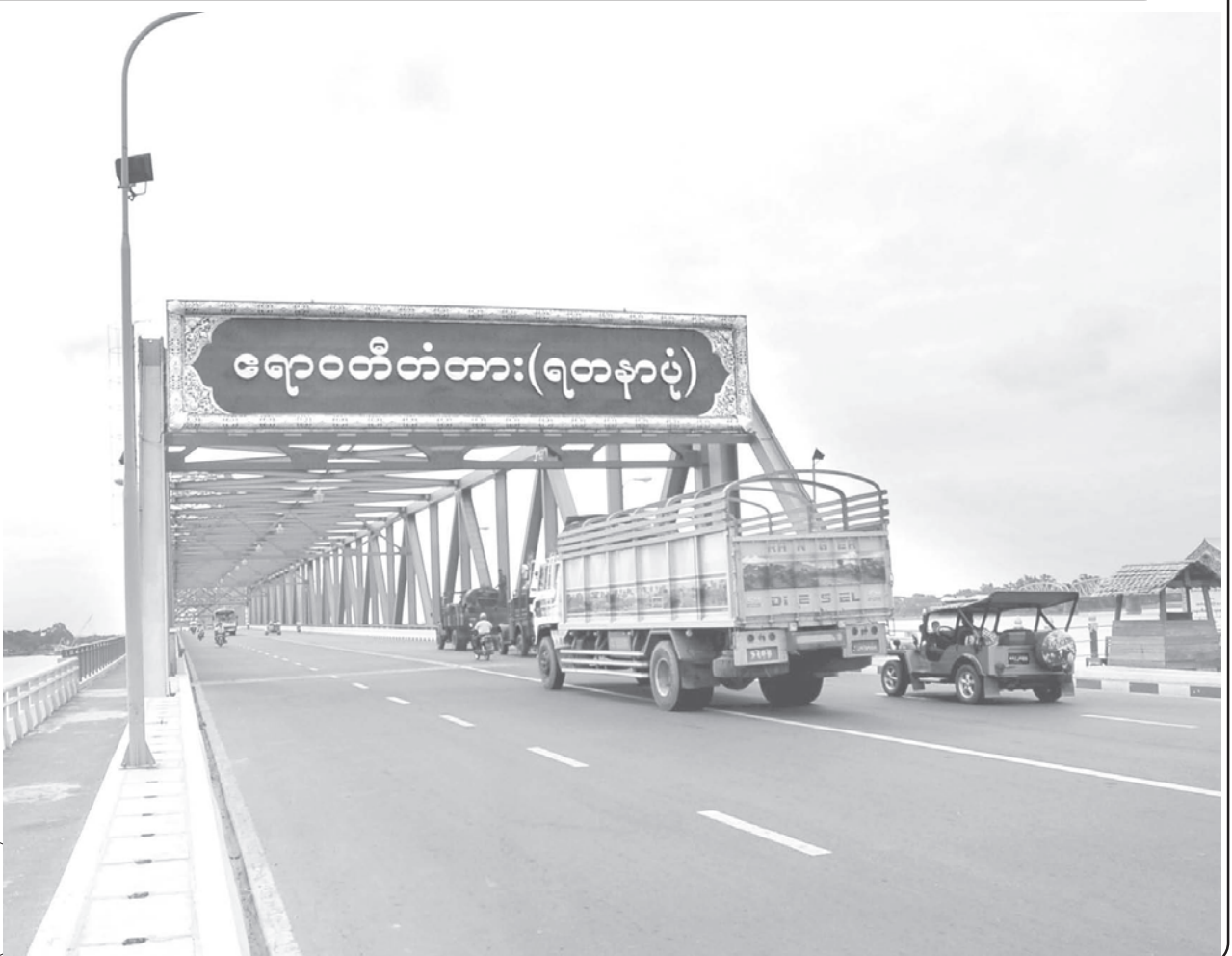
Vehicles passing through Ayeyawady Bridge (Yadanabon).
