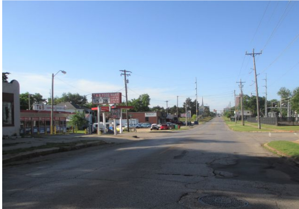
Photo C16. Overview of N. Western Avenue at N.W. 31 st Street. View facing south.
