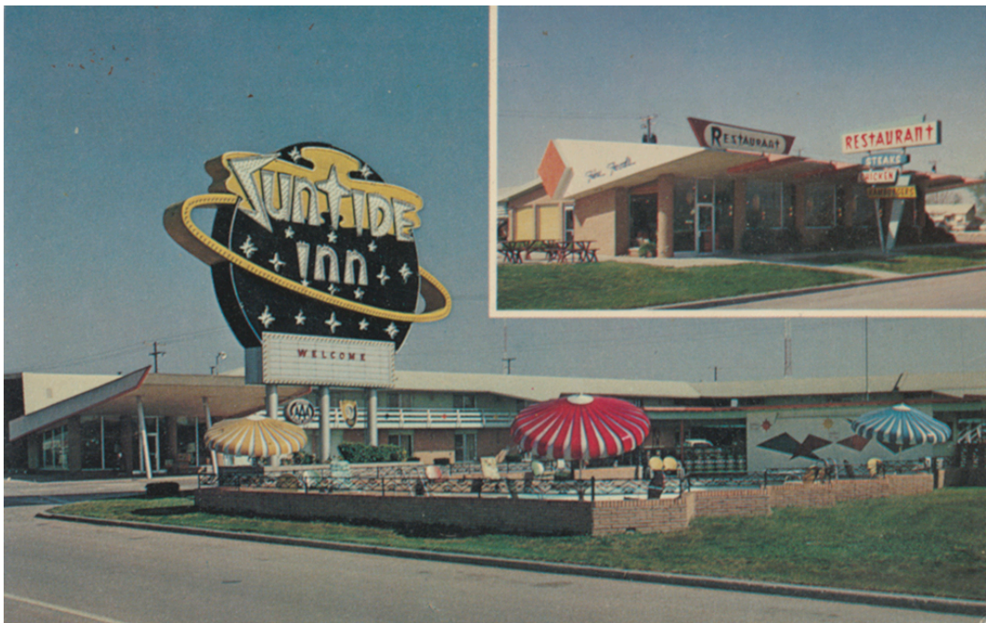
Photo B10. Suntime Inn, which was located at 3200 N.W. 39 th Street. This is an example of a typical motel from the 1960s and 1970s. Image courtesy of the Metropolitan Library Oklahoma Collection.
