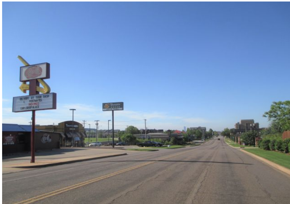
Photo C19. Overview of N. Western Boulevard near N.W. 67 th Street View facing south.
