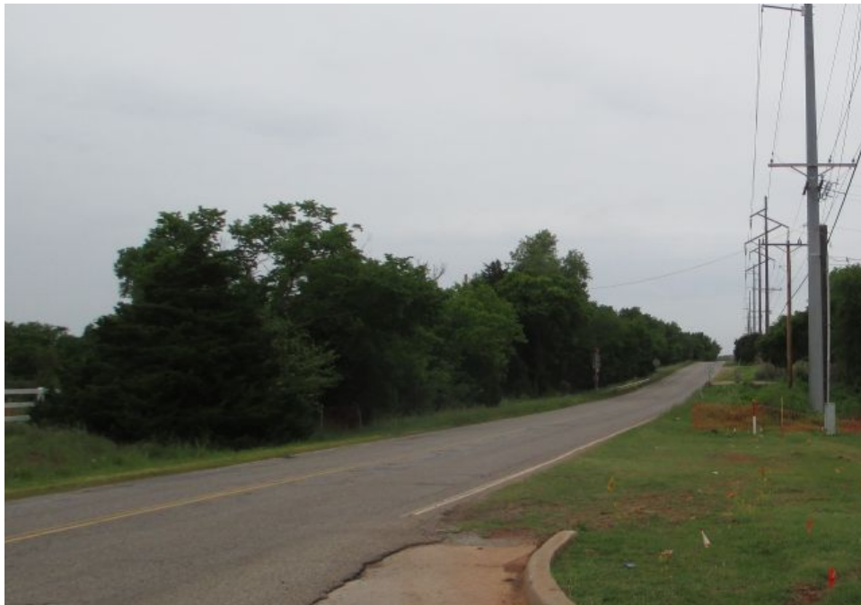
Photo C2. N. Kelley Avenue at its intersection with N.E. 101 st Street. Roadway segment maintains the two-lane without shoulder configuration of Route 66. View facing north.
