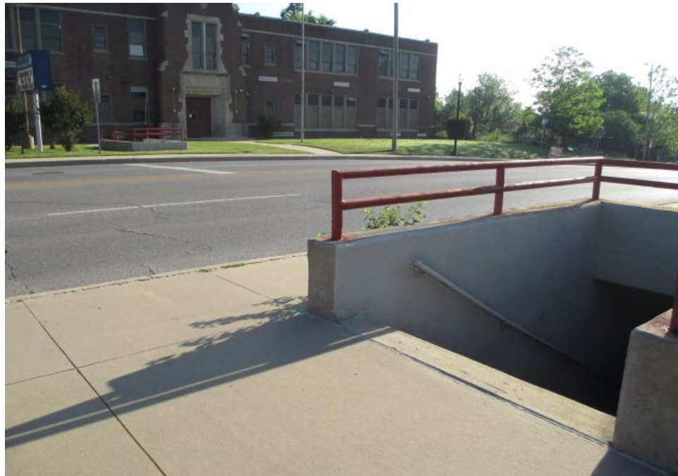
Photo C12. Pedestrian tunnel ( Resource No. 180 ) at Grover Cleveland School ( Resource No. 181 ) that has provided safe pedestrian crossing of the busy street since the 1930s. View facing north/northeast.
