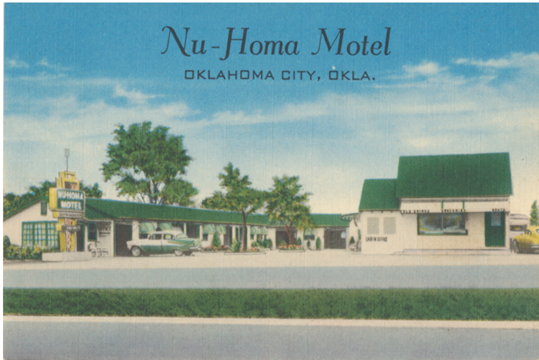
Photo B8. Nu-Homa Motel, which is located at 3530 N.W. 39 th Street, in ca. 1955. Only the office building is extant in 2020. Image courtesy of the Metropolitan Library Oklahoma Collection.
