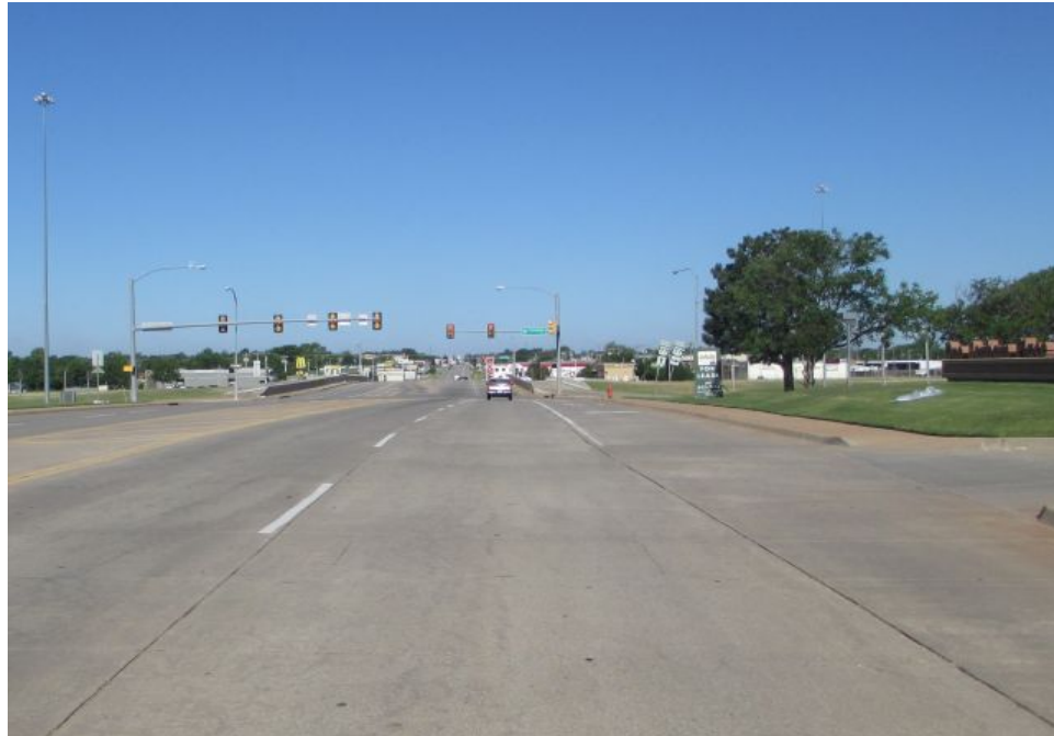
Photo C30. Overview of W. Britton Road, the former Route 66 Beltline alignment, at its intersection with U.S. Highway 77. View facing west.
