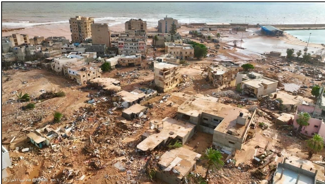
Figure 14a-b. Drone photos of the severe destruction in Derna. Source: ليبيا الأحرار / Nahel Belgherze (Twitter/X)
